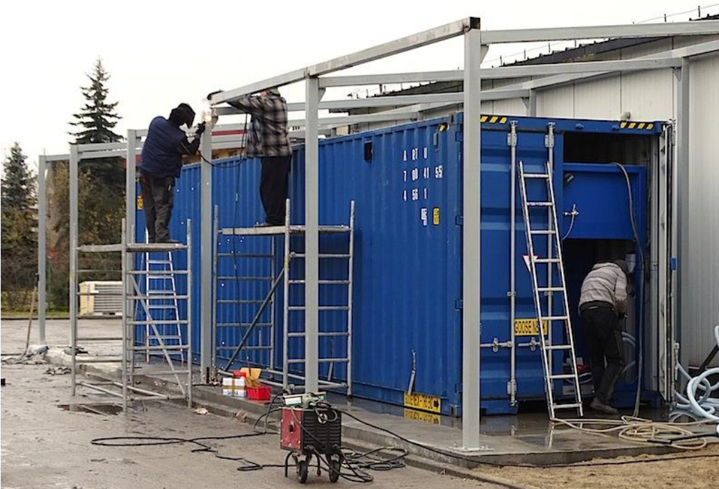
Installation of containerized plant at Polish textiles company premises
